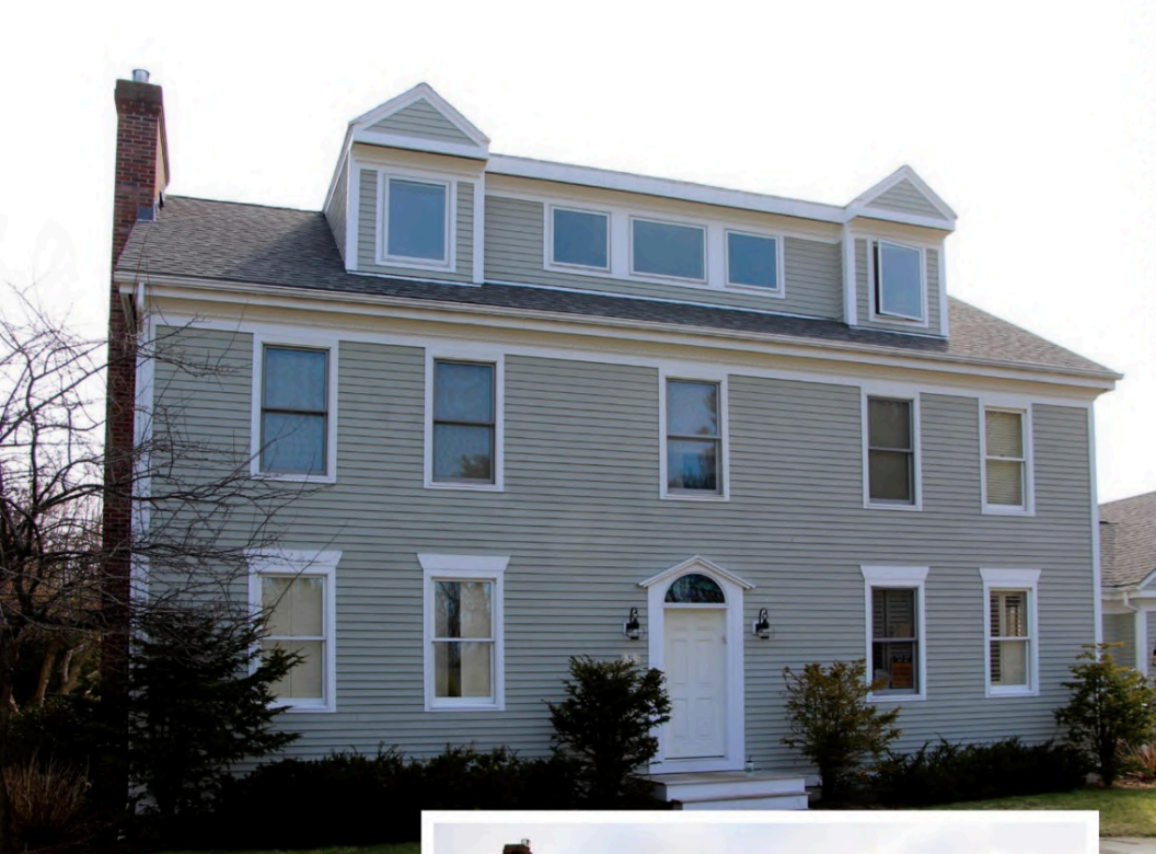
Top: After dormer addition. Right: Before dormer addition.
